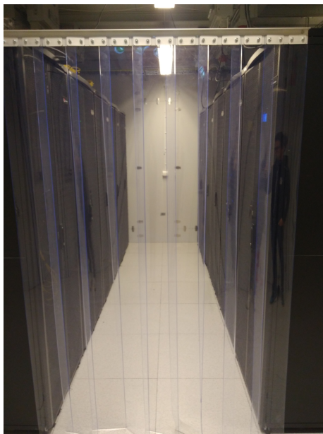
Figure 5: Photo of the hot aisle of the data center we used in our experiments.
